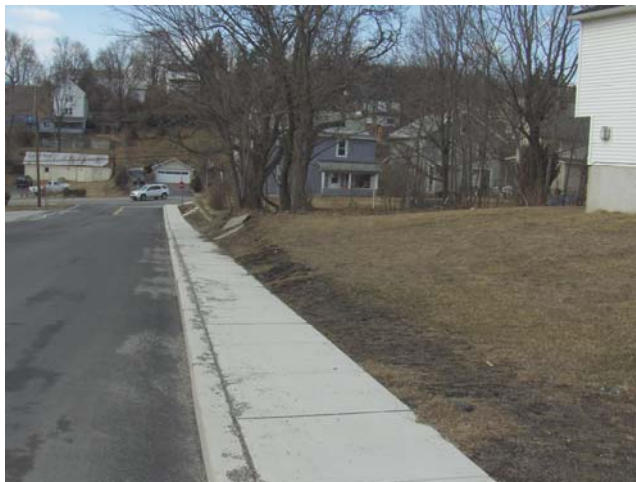
NEW SIDEWALK CONSTRUCTION
